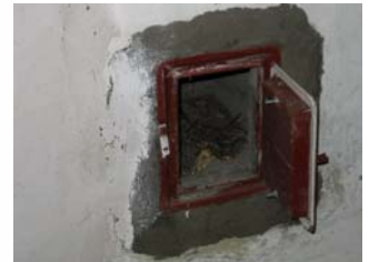
Asbest-Standard: Schnur in Revisionsklappen
